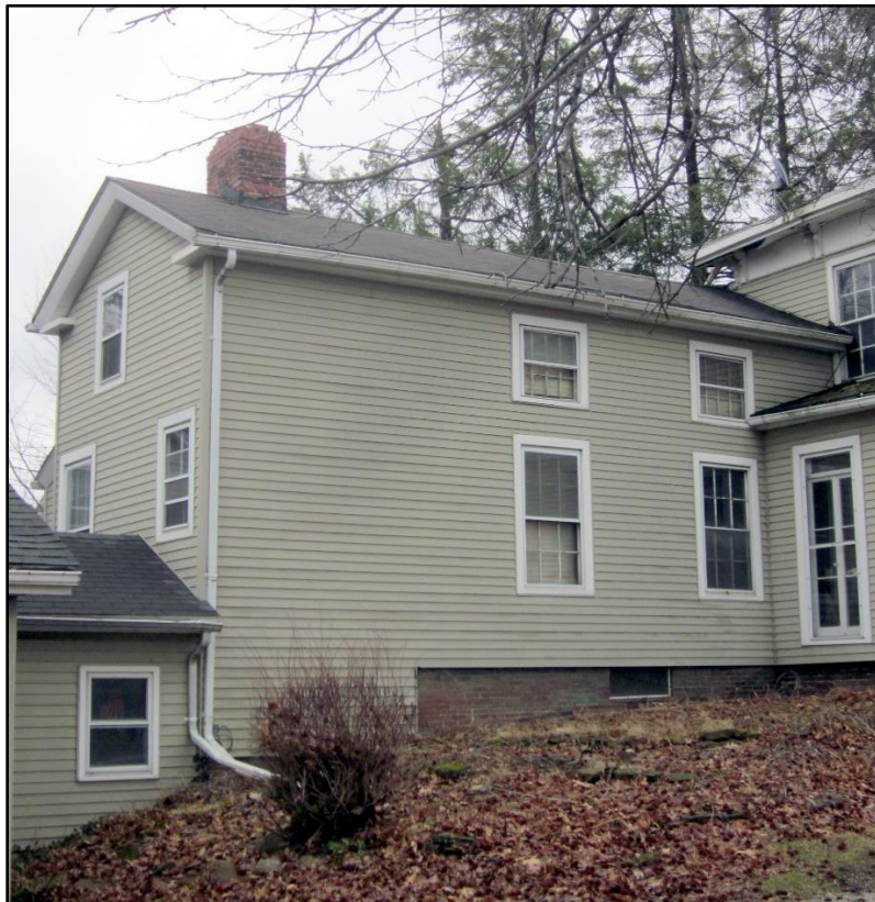
Figure 4. “The Wing,” the older part of 83 Wood Street. Only the part with the seven windows was original. An outside door to the basement was on the end, where the little breezeway is now. The basement is only under this part of the house, and the alcove, which came later, and has no entrance.
