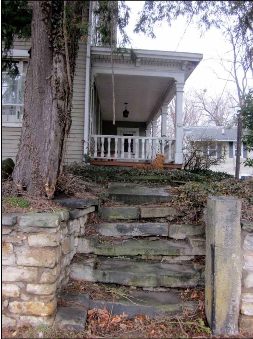
Figure 5. The original front entrance. The door has been replaced, and vinyl siding added over the original white clapboard. The iron gate is gone, and the left gatepost fell off about 1947. Photo by Cynthia Turk, 2023
